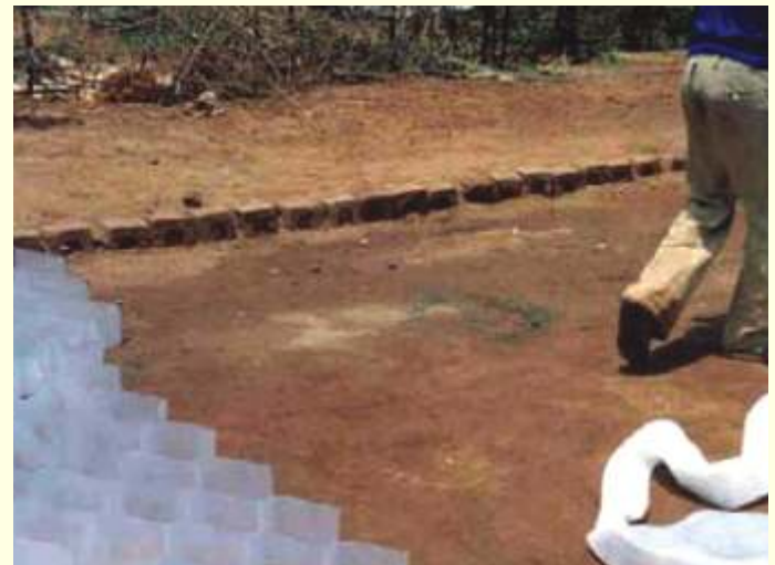
Fig 2 Formwork of plastic cell being spread
