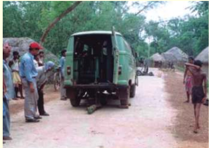
Fig 6 Evaluation of pavement by FWD
