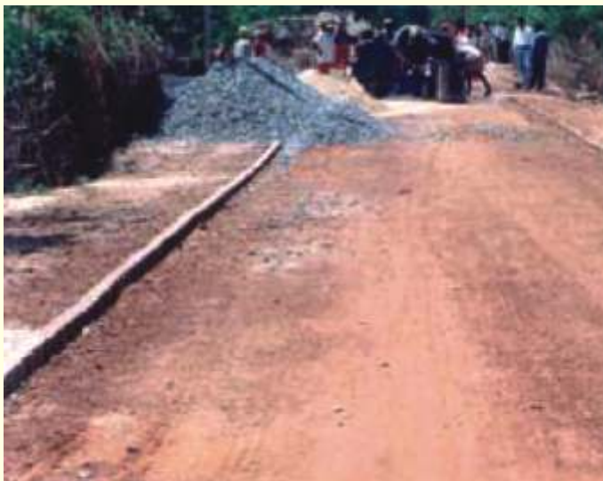
Fig 1 Murrum subbase with brick on end edge along the pavement edge
