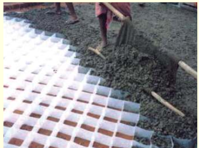
Fig.3 Placing of concrete in plastic cell
