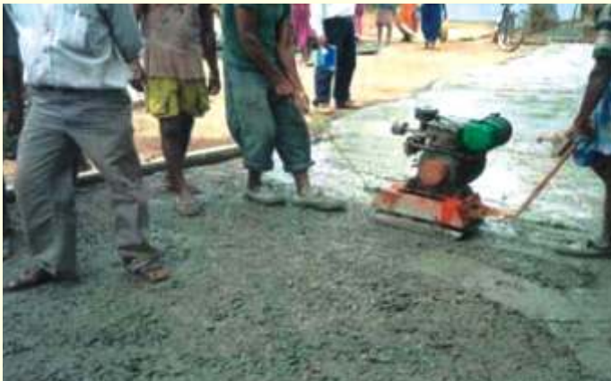
Fig. 4 Compaction of zero slump concrete by a plate vibrator
